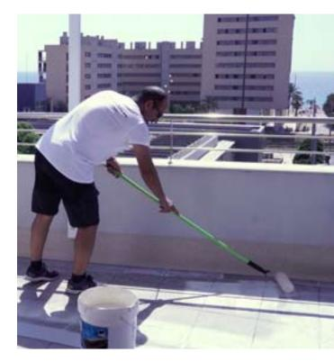
The geotextile layer is glued to the floor, making sure it coincides perfectly with the butt-welding strip, taking good care of not
