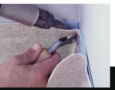
Unlike existing flooring products, the RENOLIT ALKORPLAN DECKING reinforced PVC membrane allows overlap welding, one section over another. This solution has several advantages, such as total waterproof sealing and the completion of some critical details.
