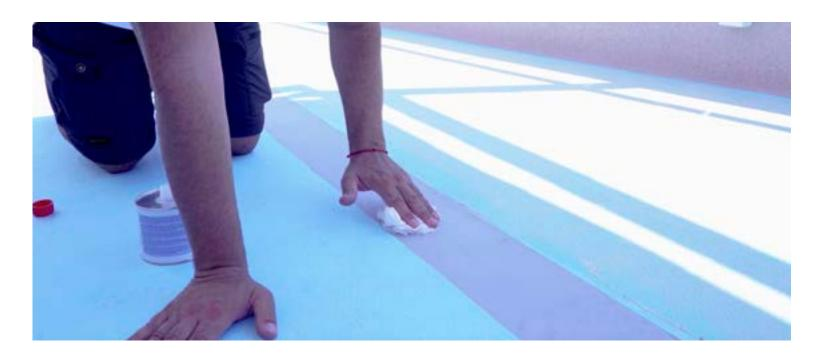
The butt-welding strips, like any other membrane already installed, can be protected with painter's tape or any other masking if needed. It is now possible to apply the membrane over the glue, taking care to position it correctly, following the installation plan. The membrane needs to be cut to size and pressed with a floor-roller to ensure its full adherence.
