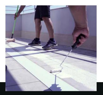
The geotextile layer is glued to the floor, making sure it coincides overlapping it, nor leaving any space between.
